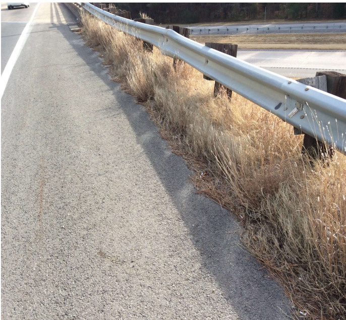
PHOTO 1 Description Impact damage to right approach guard rail & end post at Abutment 1.
