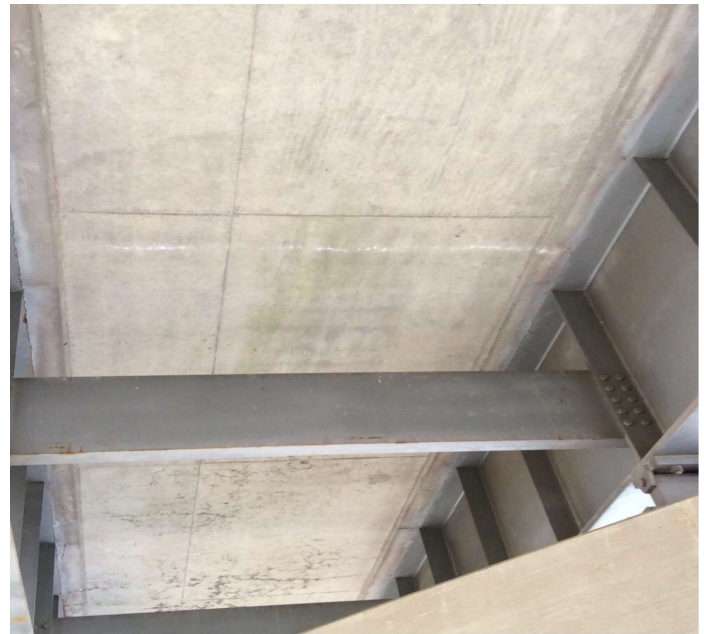
PHOTO 2 Description Typical of transverse efflorescent cracks to deck below.
