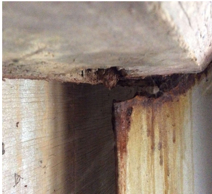
PHOTO 1 Description Hole in web of Girder 3 at Abutment 2 below paving haunch.
