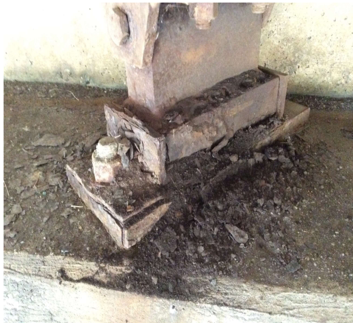
PHOTO 1 Description Rust to bearings, some with section loss Abutments 1 & 2. (G2 at Abt. 2)
