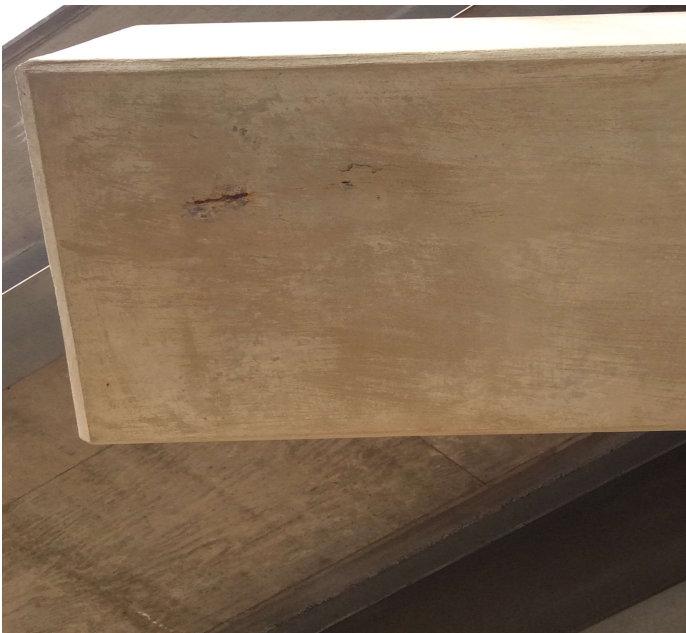
PHOTO 1 Description Spall with 3" rebar exposed to bottom right side of cap at Bent 1.
