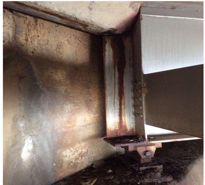
PHOTO 2 Description Hole in web of Girder 4 at Abutment 1 below paving haunch.
