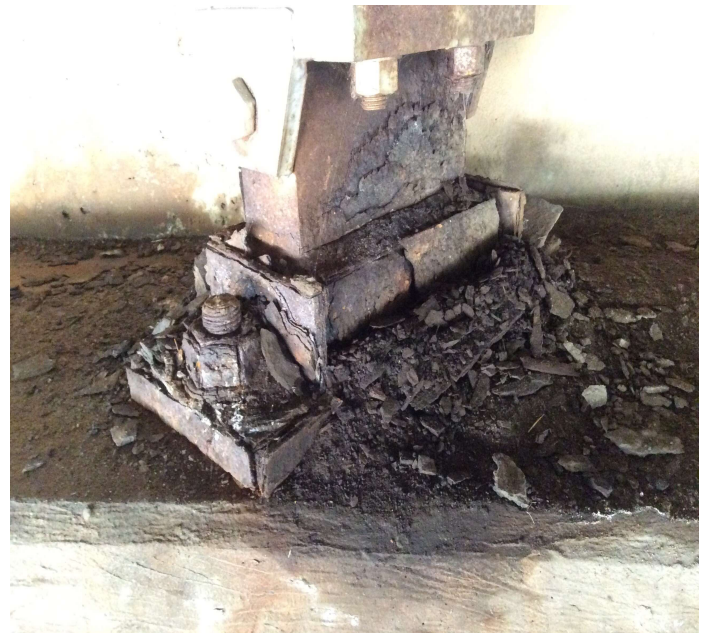
PHOTO 2 Description Rust to bearings, some with section loss Abutments 1 & 2. (G3 at Abt. 2)
