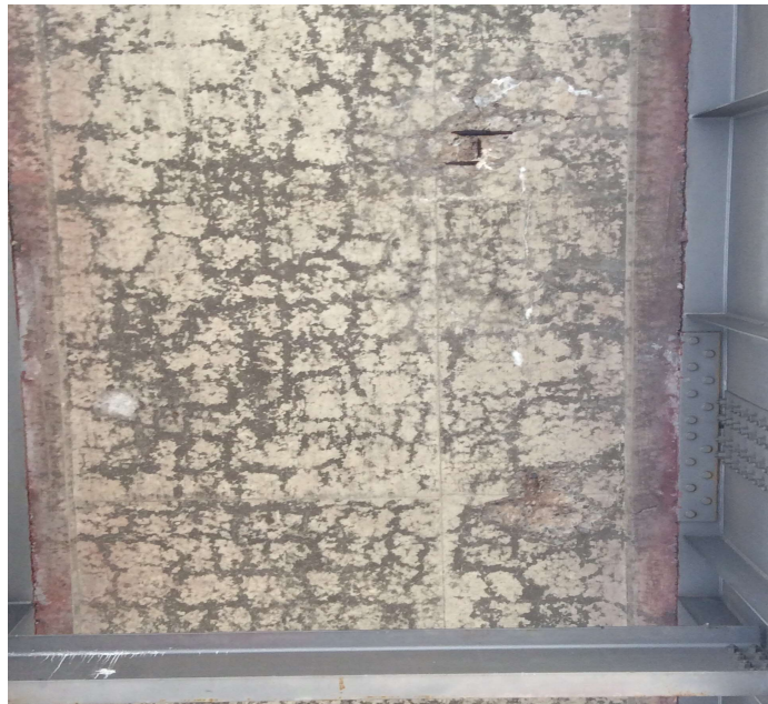
PHOTO 1 Description Typical of spalls with rebar exposed to deck below between Girders 4 - 5 at Span 3.
