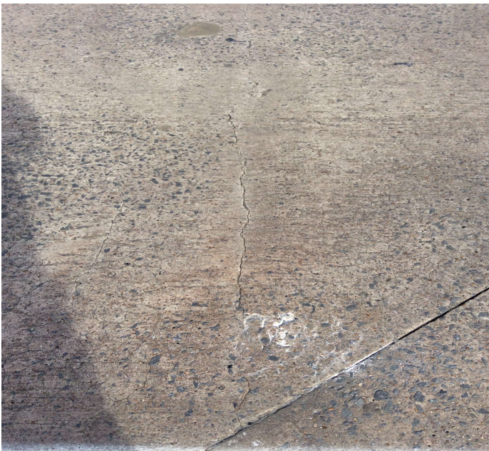
PHOTO 1 Description Unsealed transverse cracks to deck at all spans.
